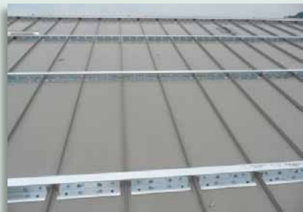
Roof Hugger sub-purlins prepared with air-circulation holes for un-insulated "ASV" application.
