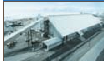
The roof of the Agrium warehouse soars up like an A-frame to meet the angle of repose of the fertilizer materials stored inside it.
