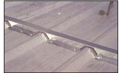
Model "C" Roof Hugger Sub-purlin System over existing 12" on center ribbed panel.
