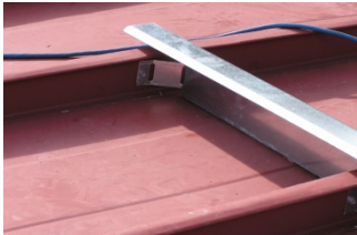
Vertical Rib Standing Seam w/ High Clips
