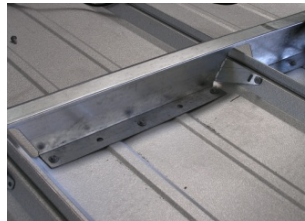
Trapezoidal Standing Seam w/ High Clips
