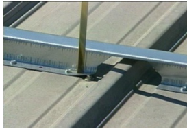
Through Fastened (Screw-down) Roofing
