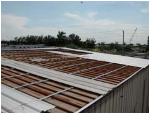
A Roof Hugger project under construction. Click image to enlarge.
