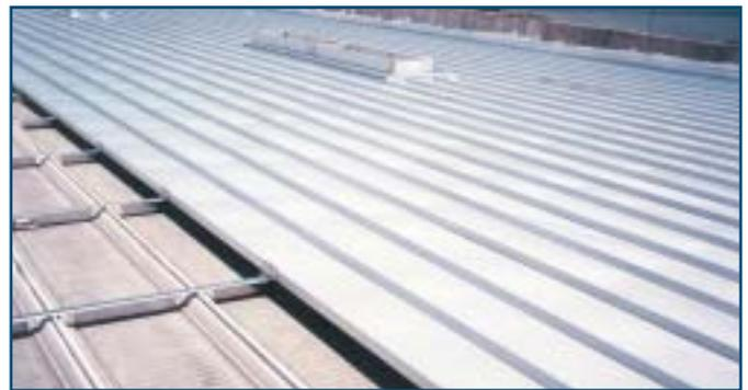
In any case, the advent of the simple, one-piece, miniature Z sub-purlin framing system has spawned a widespread and rapidly growing change in the way reroofing metal roofs is being accomplished. They present a very real and very appealing solution to an owner who otherwise faces the prospect of having to close his doors while his building is opened to the elements. That, in itself, makes the sale of a reroof the easiest sale of all.
